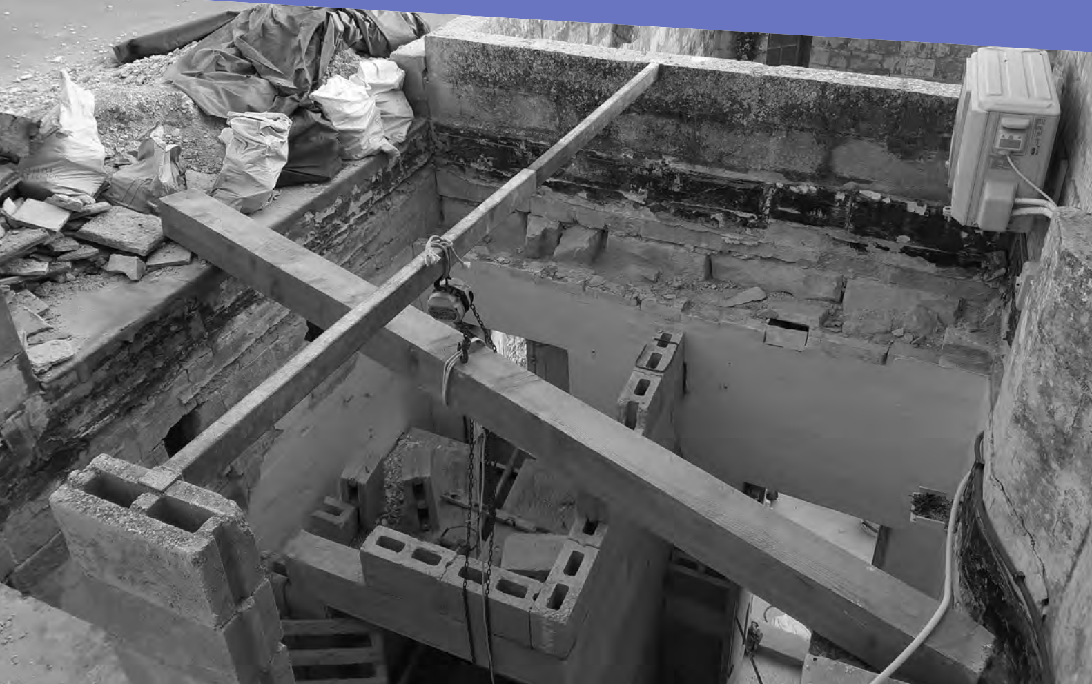
Works on the lift shaft
