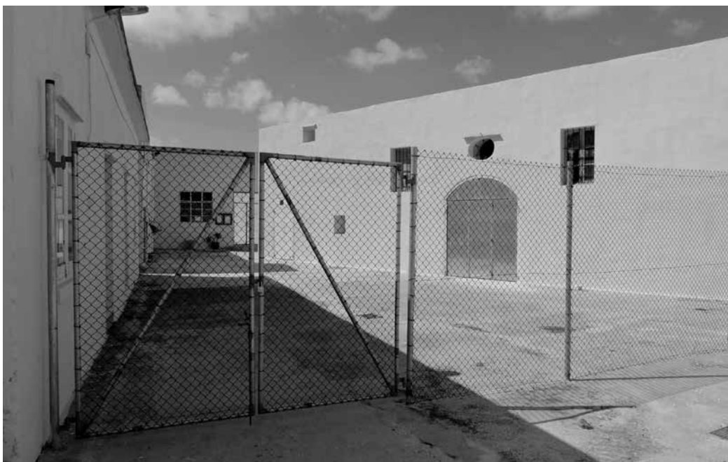
Works at the new repository at the Ospizio in Floriana.
