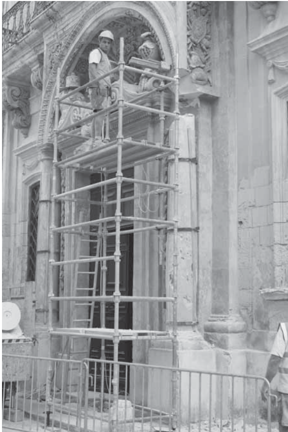
The works on the Banca Giuratale's facade
